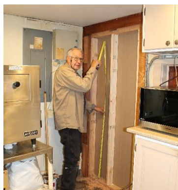
Nick Peters – Security Wiring
