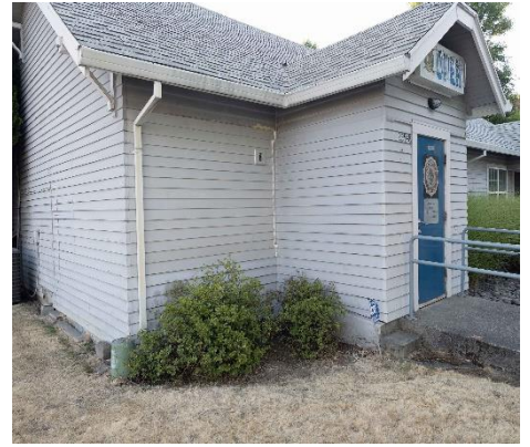
L-R: Old Boarded Up Window Replaced with New Siding – Ready for Painting
