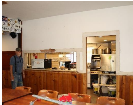
L to R Blocking up old pass-through window and old abandoned door to prep area for new cabinets and counter top
